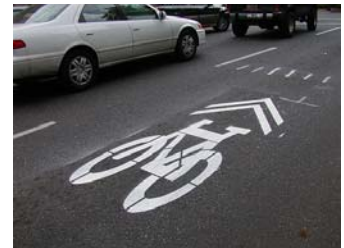
Lane markings note a “sharrow.”
